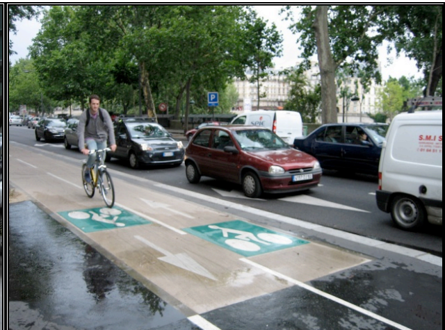
Figure 15. Contra-flow bike lanes installed where curbside car parking was removed in Paris.
